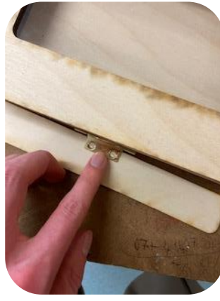
I then screwed it in using a screw driver and repeated the process for the top.
