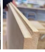
17. Here you can see the 5x5mm protrusion sticking out the shelf.
